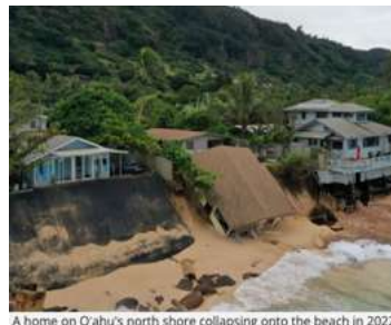
A home on O'ahu's north shore collapsing onto the beach in 2022.
